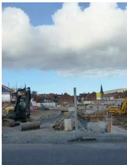
New Lodge Redevelopment
